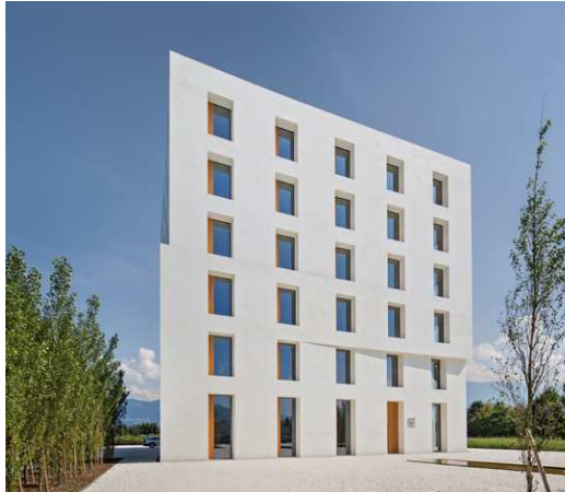
Arch. Baumschlager Eberle – Office building Lustenau (A)
